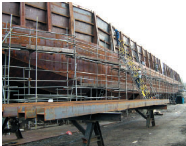
Flat Top Bridge under construction
